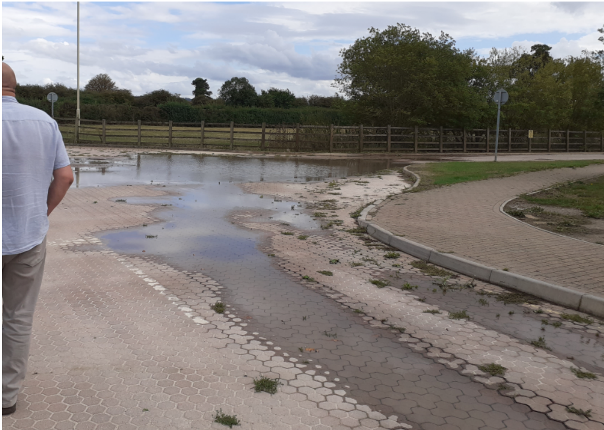
Concaving road surface from heavy vehicles – Oct 2022
