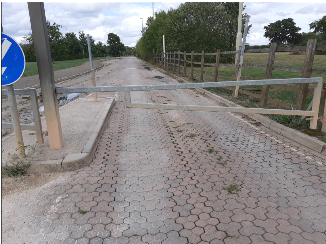
Concaving road surface from heavy vehicles – Oct 2022
